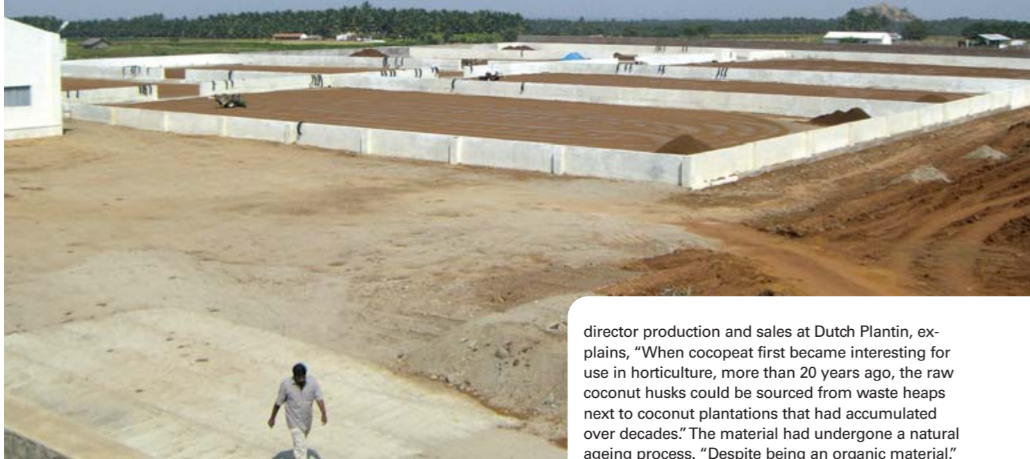
The cocopeat is dried in clean, concrete bunkers at Dutch Plantin's site in India.
